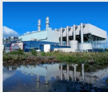
■ Damhead Creek Power Station
