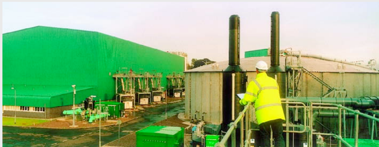
■ Above, the short stacks (right) for the ODORGARD abatement equipment and, below, the RTO units and stacks
