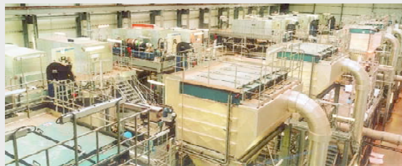
■ The Dewatering and Drying Building at Daldowie Fuel Plant
