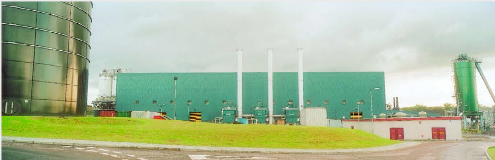
■ Daldowie's triple stacks have RTOs to treat exhaust gases
