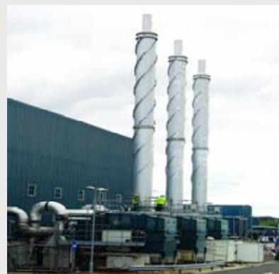
■ Above, the short stacks (right) for the ODORGARD abatement equipment and, below, the RTO units and stacks
