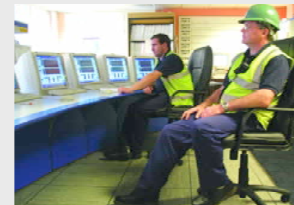
■ Monitoring production in the control room
