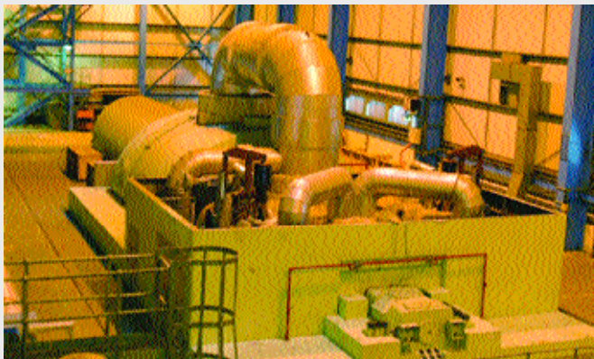
■ The steam turbine generates electricity using hot exhaust gases
