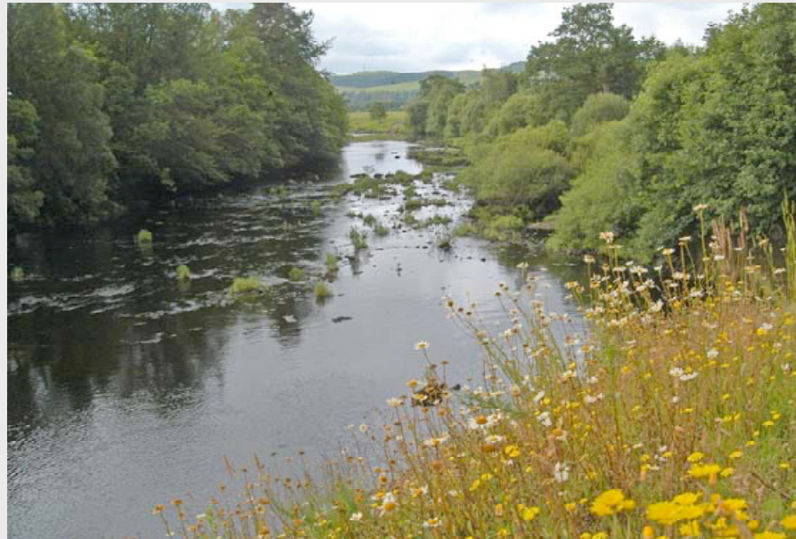
■ The outfall from Earlstoun Power Station, part of the Galloway Hydro-electric Scheme
