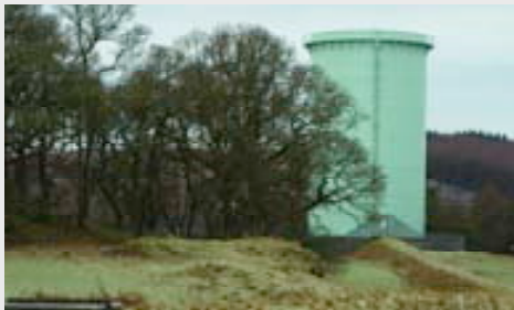
■ The Kendoon surge tower
