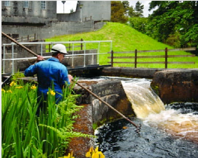
■ Clearing debris from Earlstoun fish ladder, below quality checks
