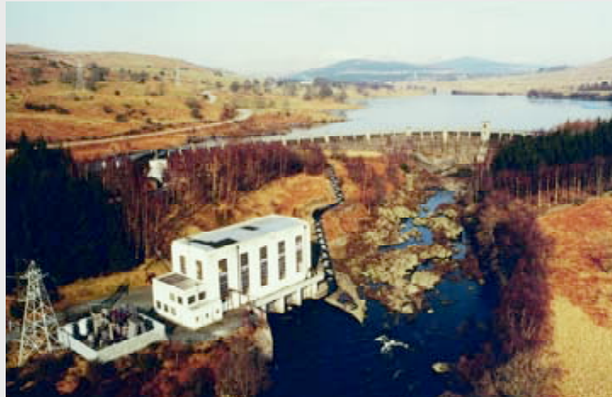
■ Carsfad, a 12 MW power station, and its 503m dam wall – the longest in the scheme
