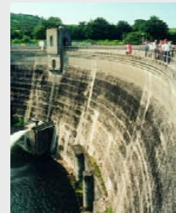
■ Clatteringshaws (left) a gravity dam, and Tongland Dam (arch and gravity)
