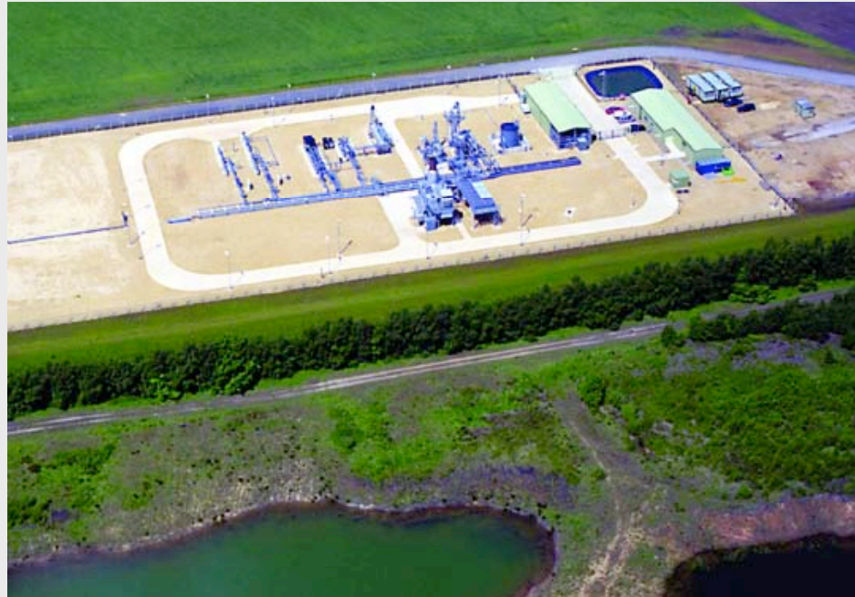
■ An aerial photograph of Hatfield Moor Gas Storage Facility’s gas compression site at Lindholme
