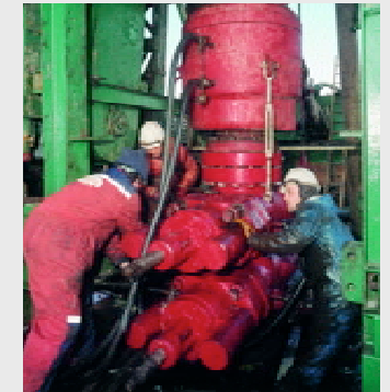
■ Construction of Hatfield Well
