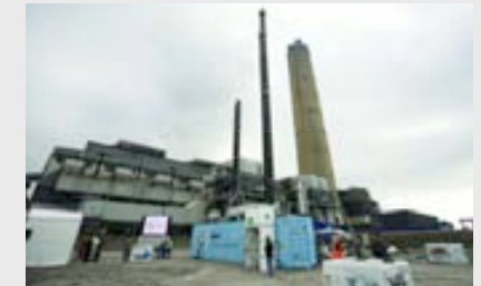
■ The MTU at its launch at Longannet
