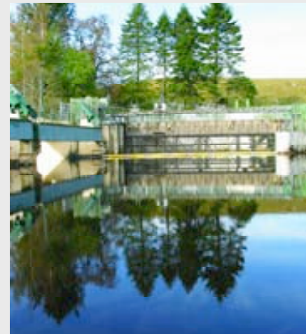
■ Work at the weir will begin this summer
