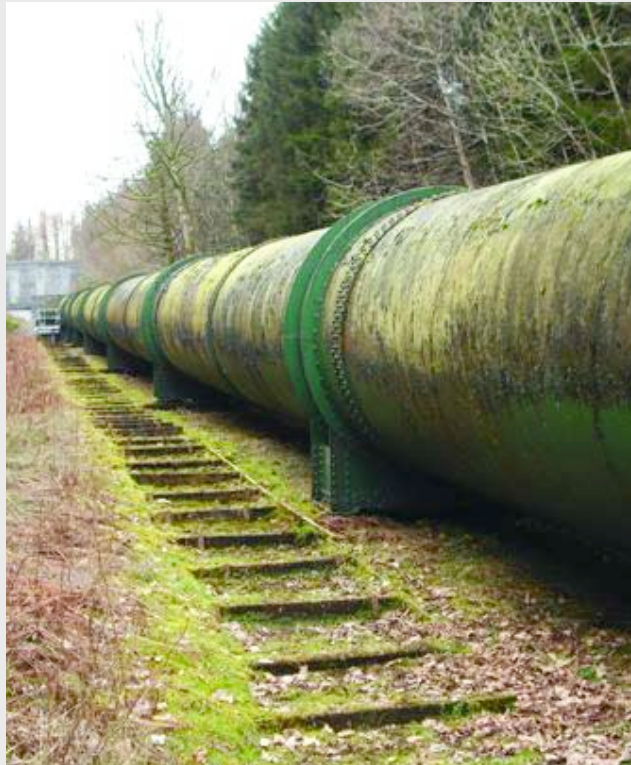
■ The Glenlee penstock (above and left), below, Glenlee Power Station
